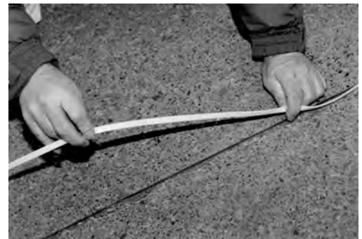
Saw Cut Loop
