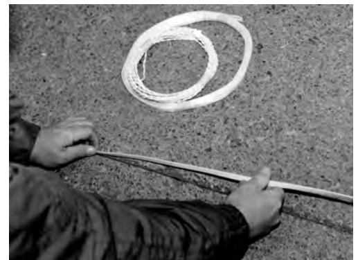
Saw Cut Loop
