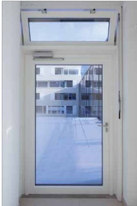
GEZE TS 5000 and OL 90 N with post-rail transmission, Nursing home Augustinum, Stuttgart, Germany (Photo: Dirk Wilhelmy)
